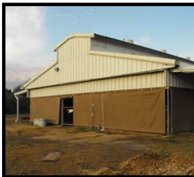
Agricultural Barn Renovations
