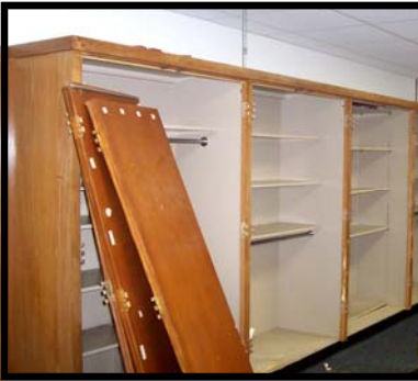
Miscellaneous Renovations / Bowie ES
