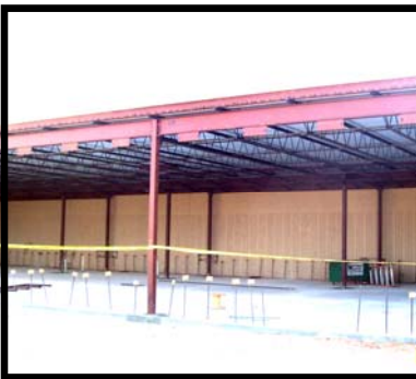
Miscellaneous Renovations / Terry HS
