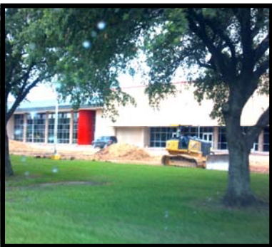
Miscellaneous Renovations / George JHS
