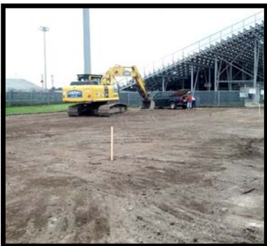
Traylor Stadium Renovations
