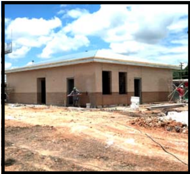
Traylor Stadium Renovations
