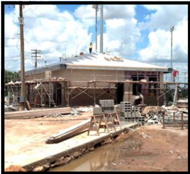
Traylor Stadium Renovations
