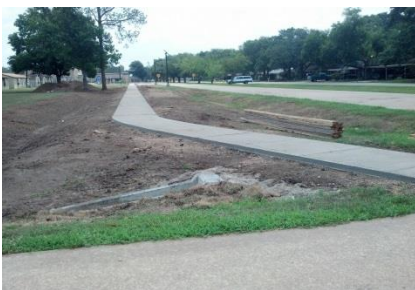
Bowie Elementary School
