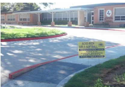
Travis Elementary School
