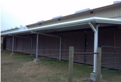
Ag Barn renovations
