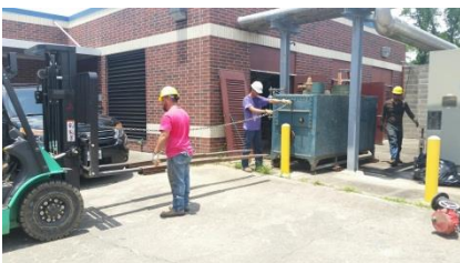
Wessendorff MS boiler removal
