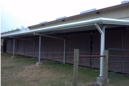
Ag Barn renovations
