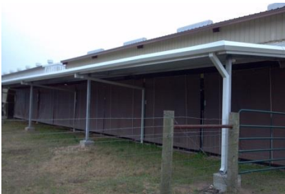
Ag Barn renovations
