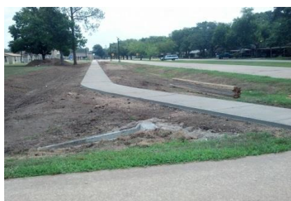
Bowie Elementary School
