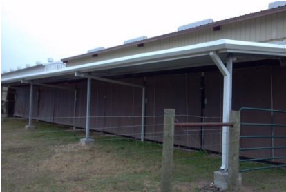
Ag Barn renovations
