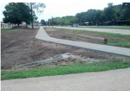
Bowie Elementary School
