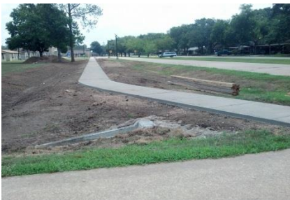
Bowie Elementary School
